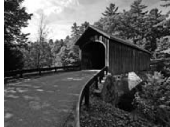
Cover inset and above: Covered bridge in Maine, USA. Photo courtesy Convention and Visitors Bureau of Greater Portland.
