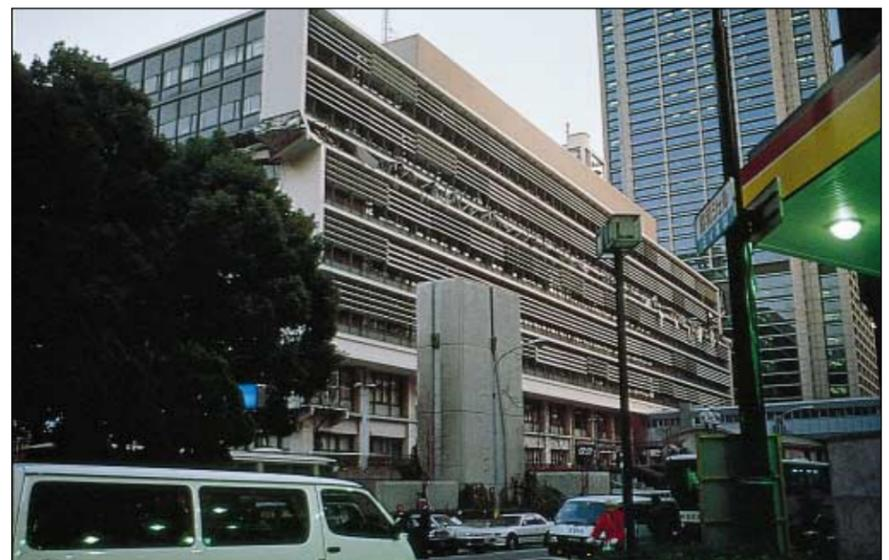
**Figure 8.** Collapsed sixth story in eight-story Kobe City Hall Annex, a reinforced-concrete building built in the 1960s. Behind it is the 16-story New City Hall, a 1980s steel-frame building that was not damaged and remained functional after the earthquake. (Photograph by Christopher Rojahn, Applied Technology Council.)
