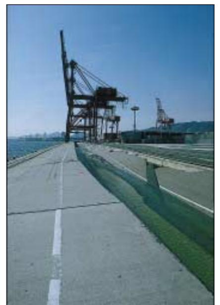
**Figure 10.** Damage to Maya Wharf caused by liquefaction-induced lateral spreading. The quay wall moved outward, causing formation of a graben. The seaward rail for gantry cranes is located on the quay wall, and the landward rail is located on a pile-supported wall behind a graben.
