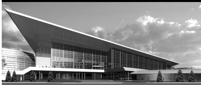
2004 Expanded Colorado Convention Center. Image used with permission from Denver Metro Convention & Visitors Bureau.
